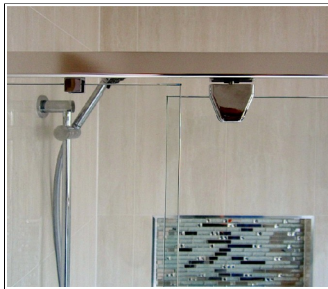
The Shadow door pivot shown with minimal top clamp for sidelite panel
